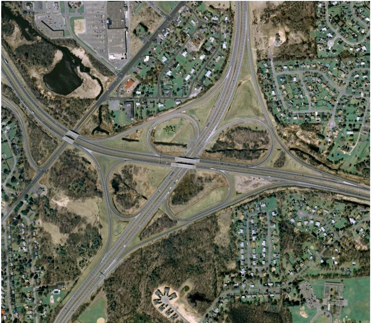
I-81 & I 481 Interchange, North of Syracuse
